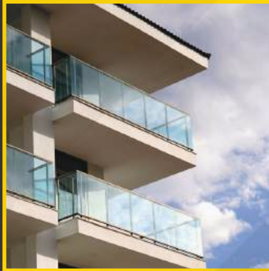
Building Construction Bauindustrie
